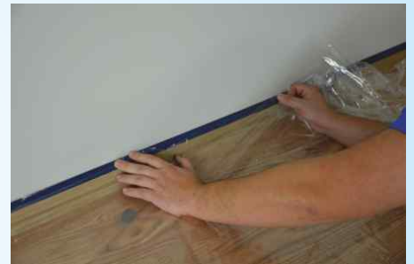
Apply dust sheet directly over tape
