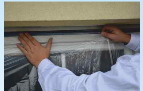
Apply dust sheet directly over tape
